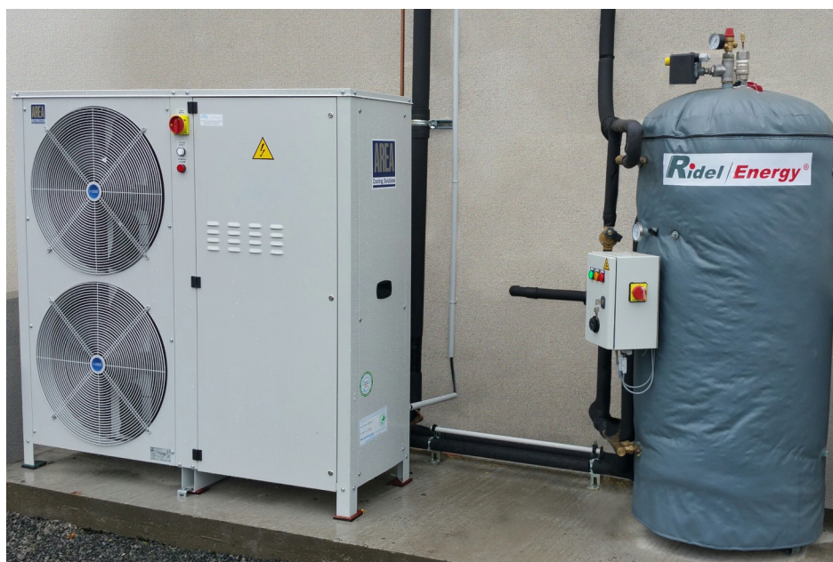
Icool Unit– PTXISS 21D HP / Rejection power = 20 kW
